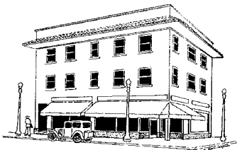
The Stevens Building
